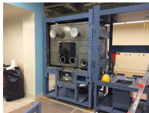
Chamber of the cell for producing Tc-99m is installed.
